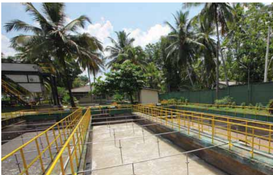
Effluent treatment plant, Ceylon Cold Stores, Ranala
