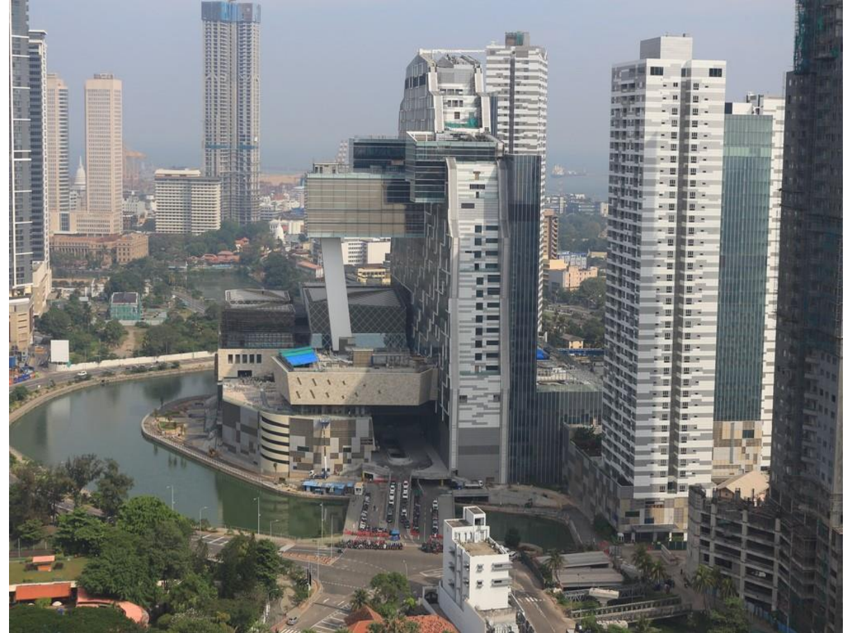
Actual construction of “Cinnamon Life” as of January 2023
