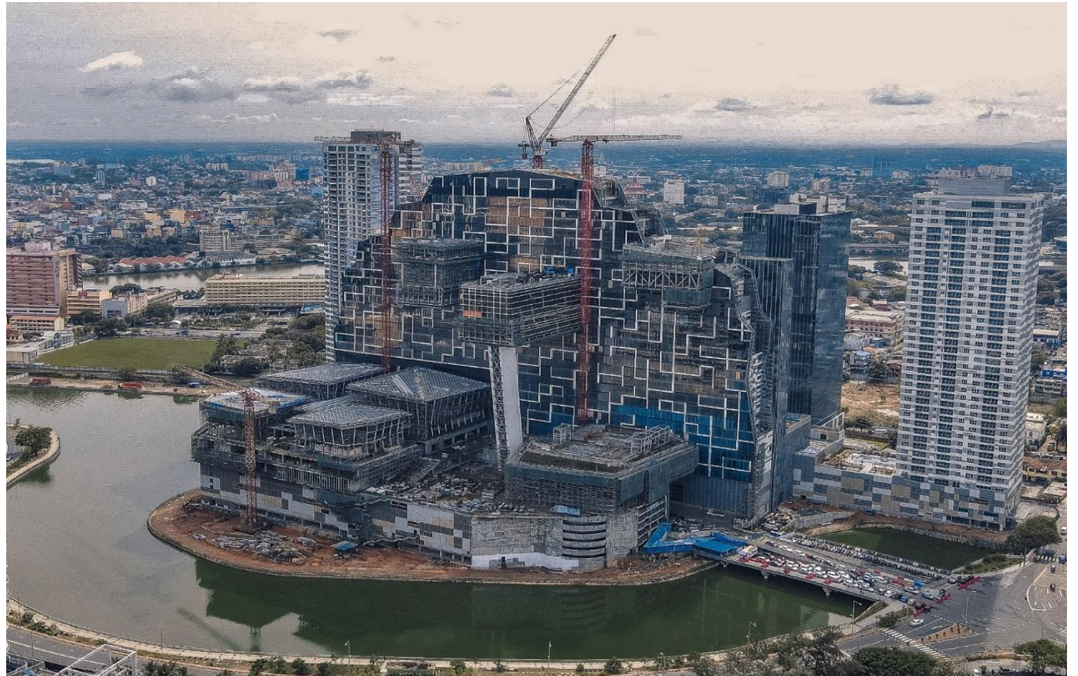
“Cinnamon Life” under construction
