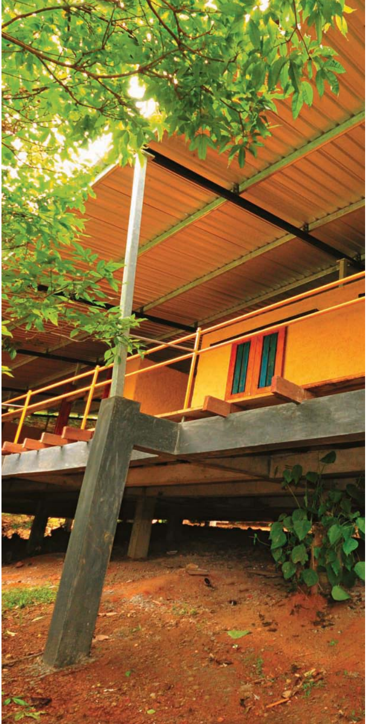
The Rumassala Nature Field Centre developed in conjunction with the Central Environmental Authority; a first of its kind in Sri Lanka
